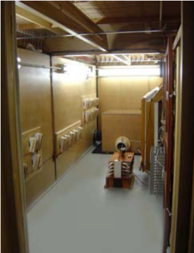
Interior of the Airbox. This “room” stands 5’ above the floor, allows complete access to the blower, D/C rectifier, solid-state switching system, Austin-patent concertina-style swell motor (center) and of course, all pneumatics, manual pneumatics (top) and Pedal Open Diapason (along wall at left).
